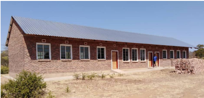
A triple classroom block, Dambwamukulu Secondary School
